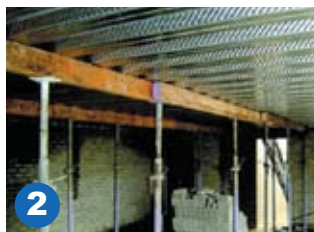
Place temporary support if required
