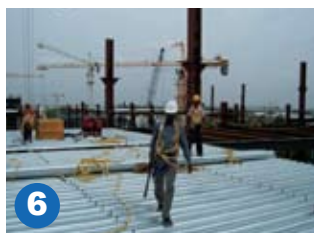
Fix SMARTDEK™ 51 profiles to steel or concrete beam
